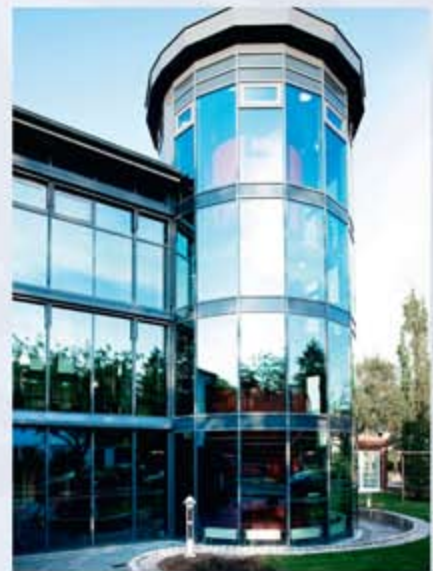
Office Building Wandsbek, Hamburg / Germany
