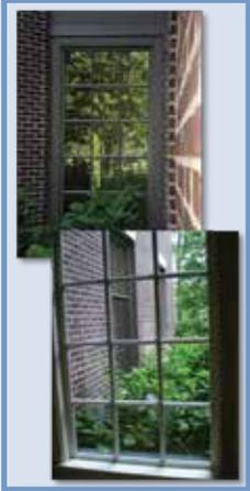
For this project, the homeowner retrofitted one window in 2009 with first generation ORNILUX SB1 as a trial to see its effectiveness in preventing window collisions. Pleased with its performance, in early 2011 the homeowner retrofitted a second window with ORNILUX Mikado.
